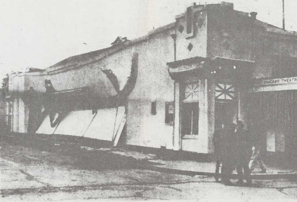
The walls of the Port Chicago theatre were blown in by the force of the blast
