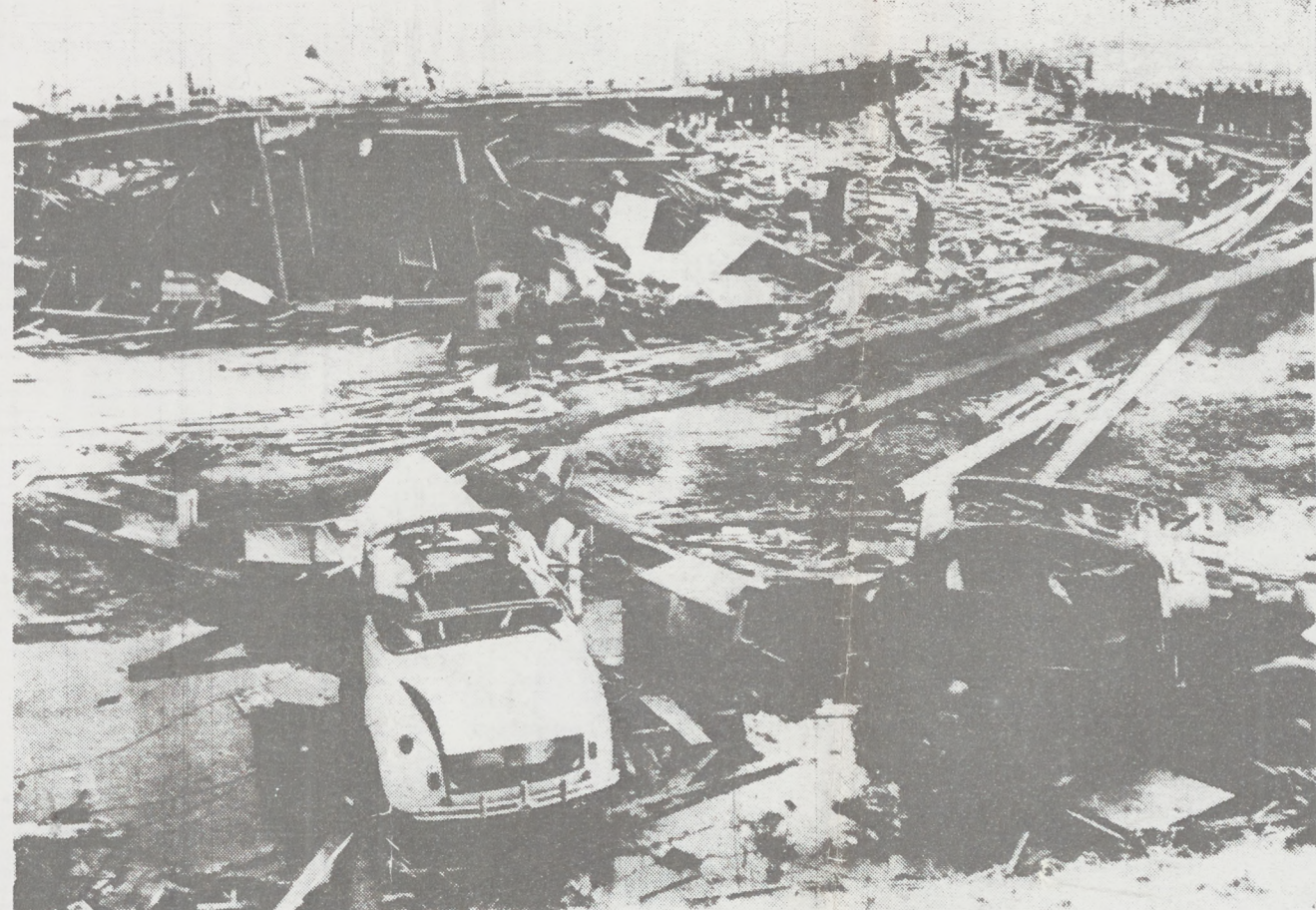
Automobiles parked near the dock area of Port Chicago, Calif., were blown apart. In the background are the ruins of one of the docks
