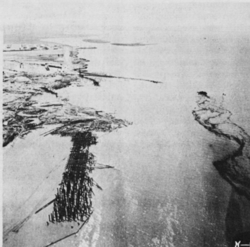
View of destroyed main pier and marginal pier (foreground), which was under construction at time of explosion. U.S. Navy photo.
